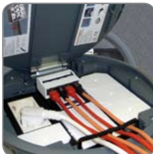
Installation in floor box
